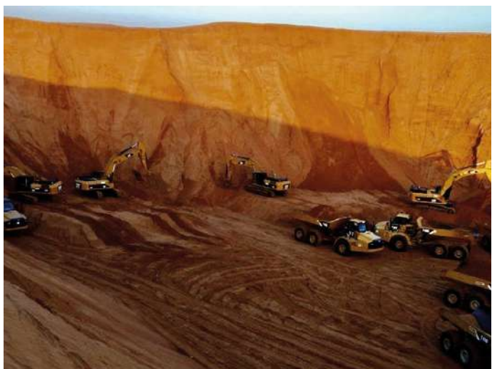
Dune Sand Filling Mountain Slope Protection Dune Sand Excavation
