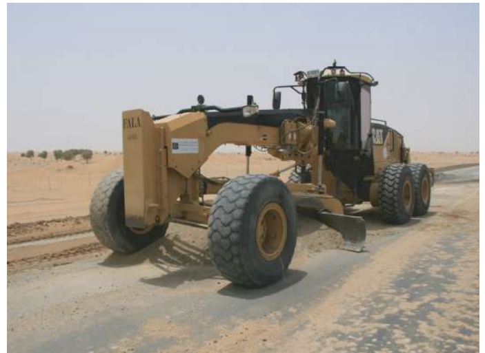
Road Base Mixing Sub Base Laying
