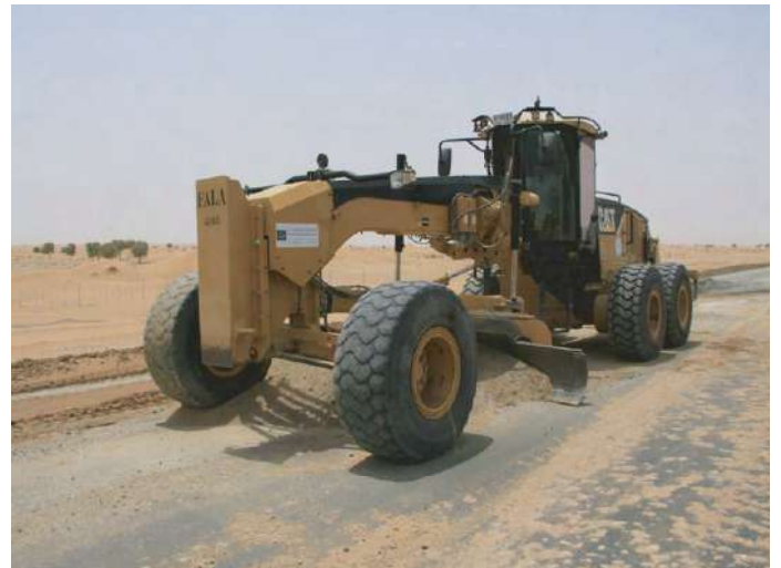
Road Base Mixing Sub Base Laying
