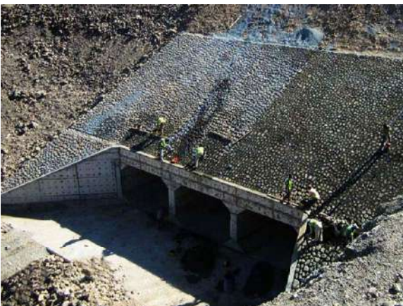
Bridge works Pipe Culvert Works
