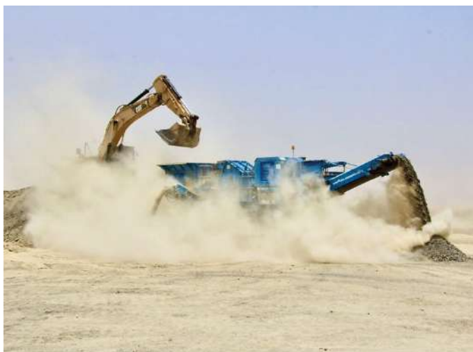
Road Base Laying with paver Screening & Material Crushing
