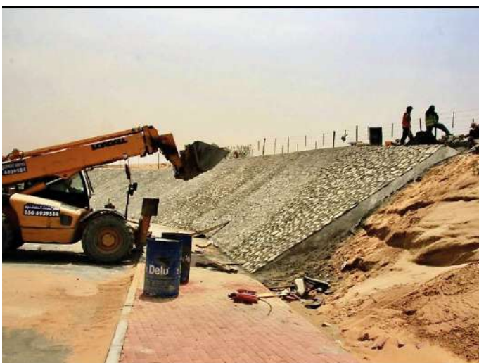
Asphalt Compaction New Jersey Barrier Cast in Situ Rip Rap Protection Work
